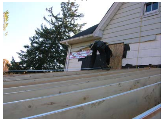
Picture 4: Applying the tape with two people.
