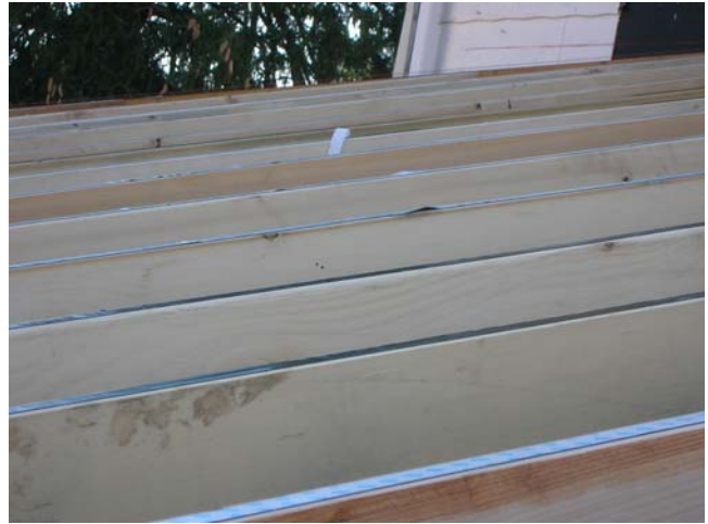
Picture 6: Some rafters with tape still protected and others with the protective paper already removed.
