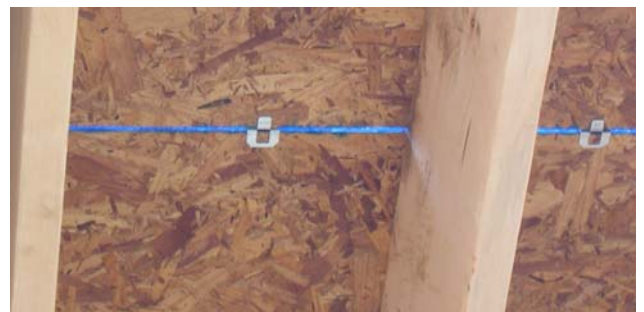
Picture 7: H-clips with sheathing panels installed.
