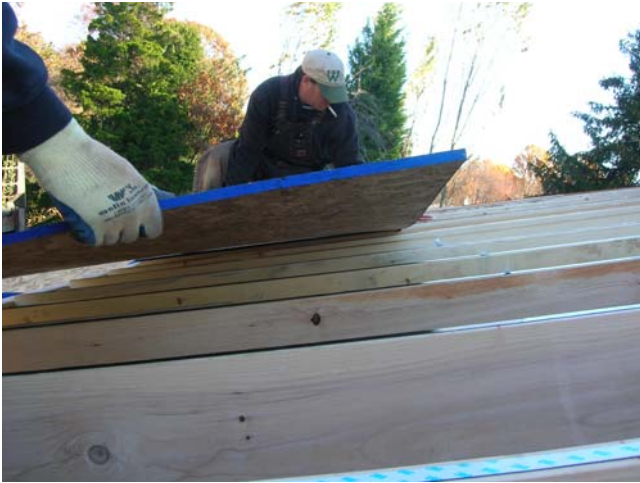
Picture 5: Crew installing the first sheathing panel.
