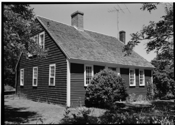
Figure 8 - Cape cod house from U.S. Library of Congress survey of historic houses
